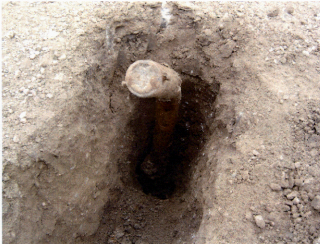
Position of pipe established by excavation.
